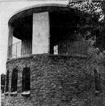
INFIRMARY PORCH—This is a view of the porch of the infirmary, which is part of the newly constructed wing of the monastery. The porch overlooks the monastic enclosure.
