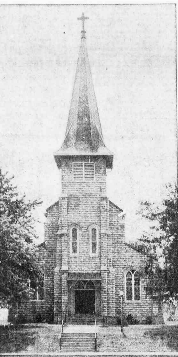
TO OBSERVE CENTENARY—St. John's Church, Starlight.
