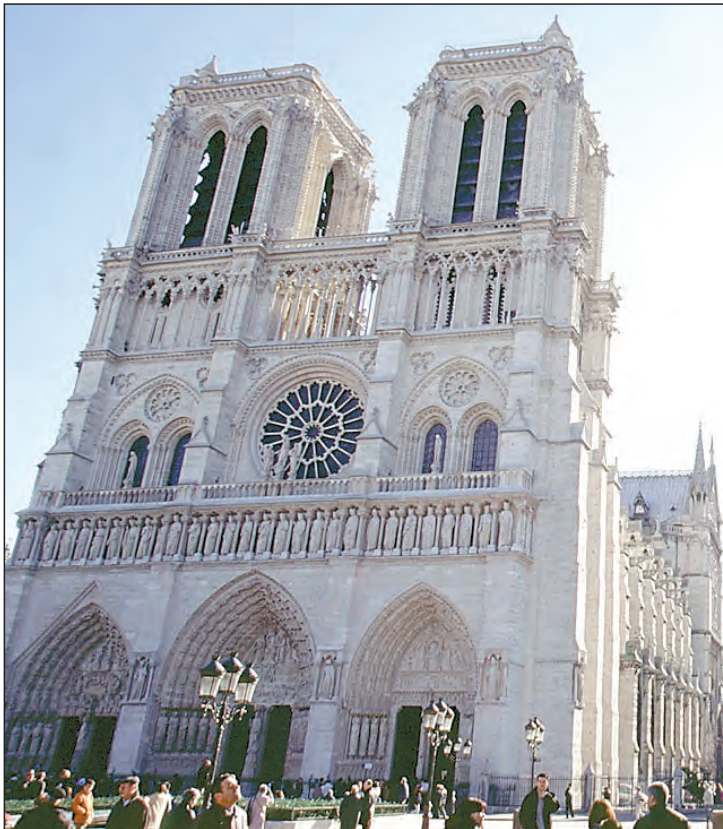
The front facade of Notre Dame Cathedral is pictured following a five-year restoration project. The cleaning, which used high-tech and biological processes, has brought out details in the Gothic sculpture that had been covered with hundreds of years of grime. Left, a gargoyle high up on Notre Dame Cathedral peers over the city of Paris.
