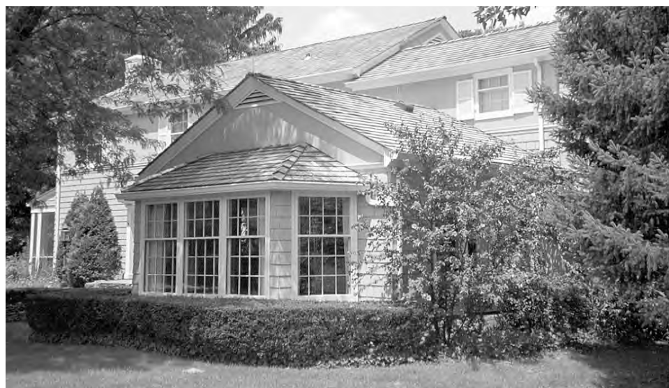
Roof Certified by Cedar Shake Bureau—Labor and Materials #1 Grade Red Cedar Shingle with Copper Flashing
