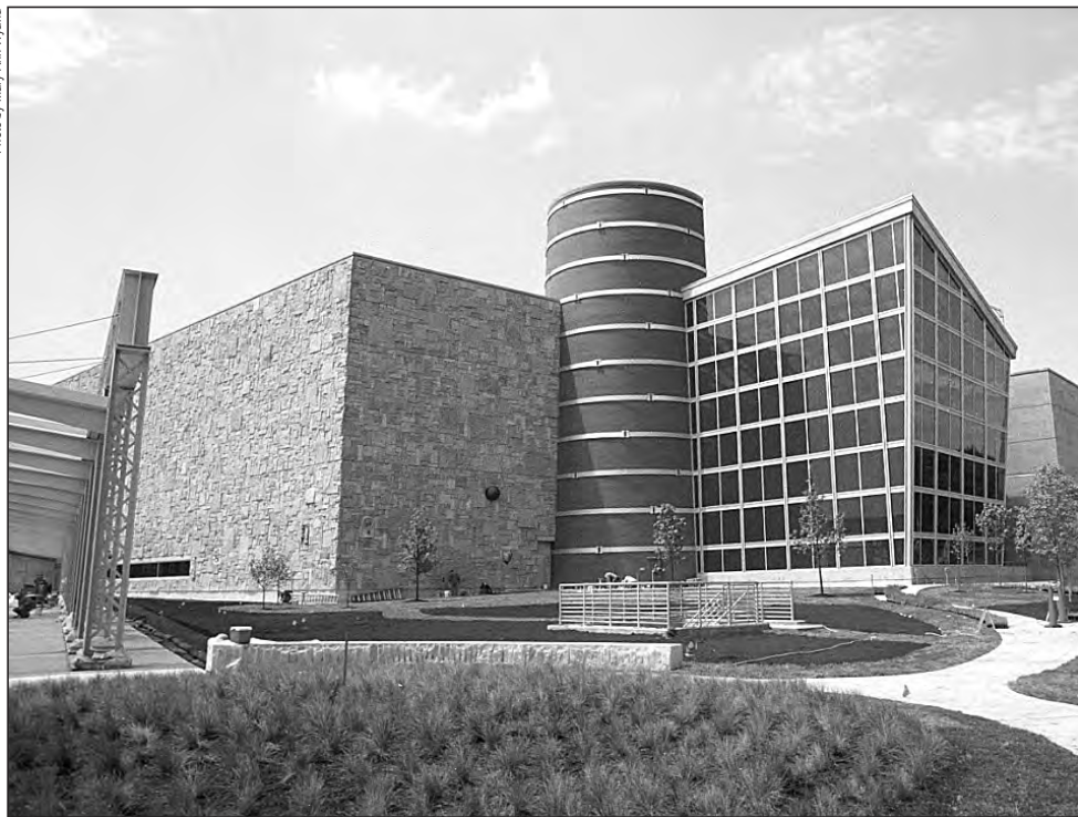
Construction and exhibit work continued in early May on the new Indiana State Museum at White River State Park in Indianapolis. The museum was dedicated on May 22 and is now open to the public. The museum features a new sculpture titled "Indiana" created by noted Hoosier artist Robert Indiana.
