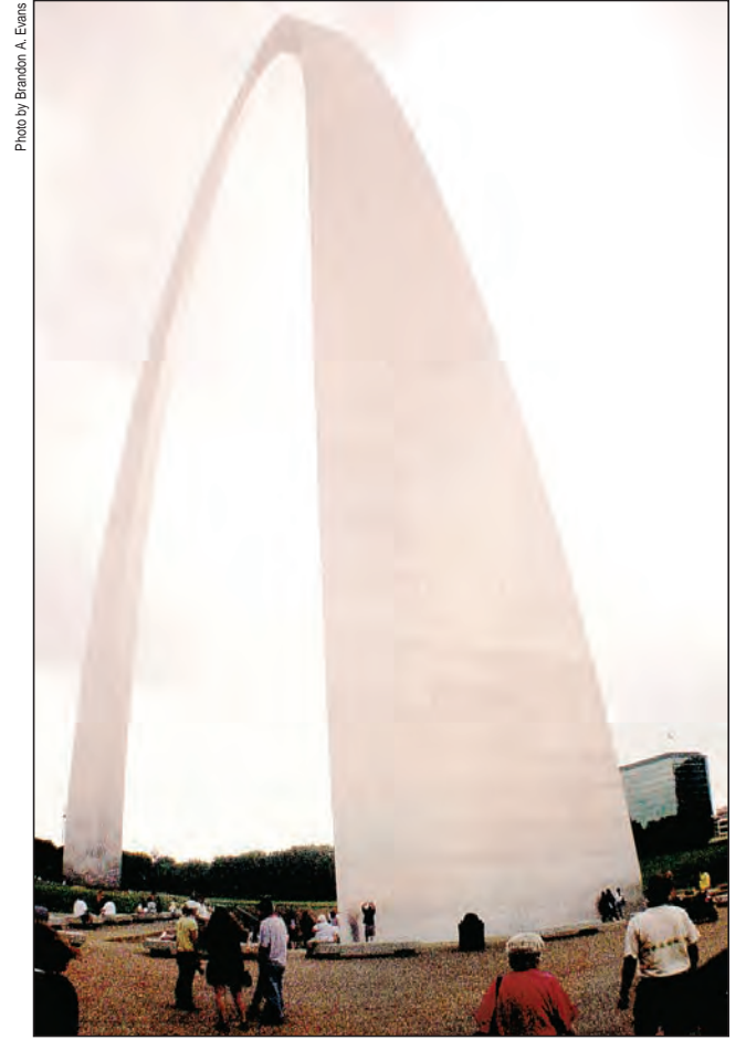
Tourists approach the Gateway Arch at the Jefferson National Expansion Memorial Park on the western bank of the Mississippi River in St. Louis last summer. The stainless steel Arch is 630-feet high, has a 60-foot foundation and features a small viewing area with windows that is accessed by small groups of passengers riding a tram-style elevator. The weighted catenary curve was designed by architect Eero Saarinen in 1947, built between 1961 and 1965, and dedicated in 1966. The nation's tallest memorial commemorates the westward expansion of the United States. The Underground Visitor Center includes a museum, theater and gift shop. The historic Old Cathedral, originally a log chapel built in 1770, is near the Arch.
