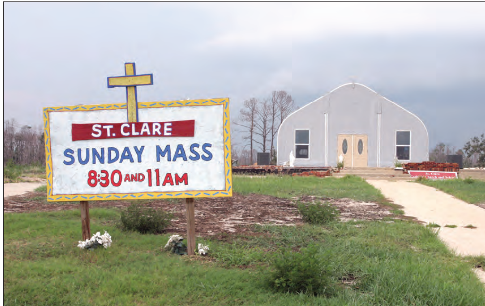
A sign displays the Mass times at St. Clare Church in Waveland, Miss., where the parish currently conducts services in a donated Quonset hut on the concrete slab where the church once stood. The Diocese of Biloxi, Miss., was hit hard by Hurricane Katrina on Aug. 29, and steps have been made toward recovery, but full-scale recovery is still a long way off.
