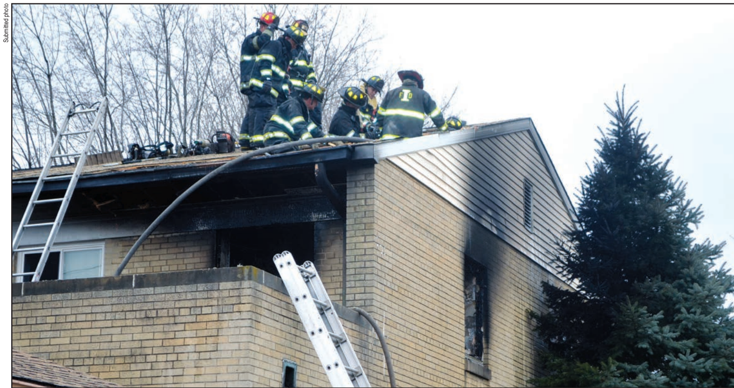
The Indianapolis Fire Department responded to a fire at the convent of St. Bernadette Church in Indianapolis on Feb. 28. The fire is believed to have been accidentally started from a burning candle. Firefighters had the fire under control within 30 minutes.
